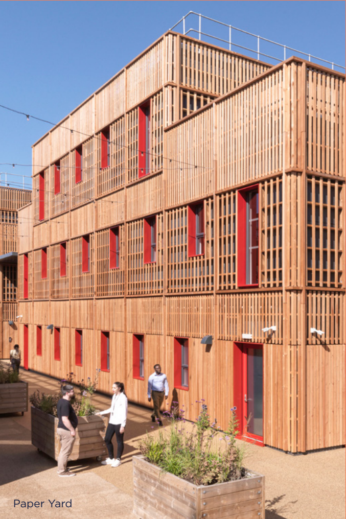
The Paper Yard is composed of lightweight, reusable modules that can expand over time. The light structures also save on foundations, and modular assembly cuts construction waste by up to 90%.
